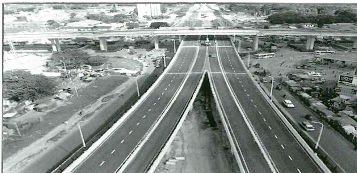
Photo 3.8.1: Ubungo Road Interchange nearly completed June 2020
