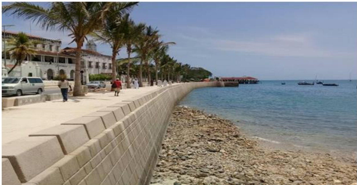
Picture 3.3: Mizingani Seawalls constructed at Forodhani, Zanzibar
