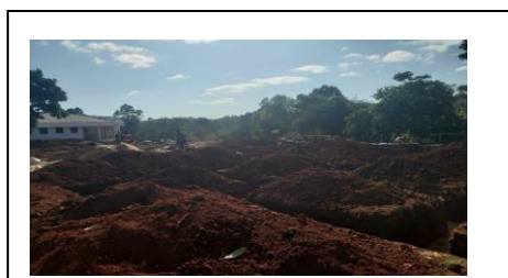
Figure 14: ICU Construction at Mbulu Town Council
