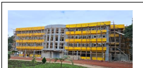
Figure 23: Classroom, lab and offices at ATC
