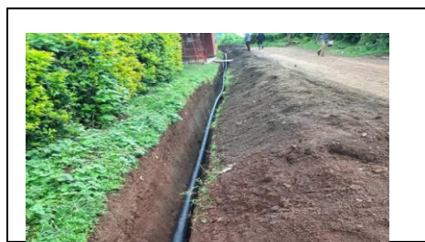
Figure 17: Figure 18: Pipe laying Kimochi – Moshi DC Hanang DC
