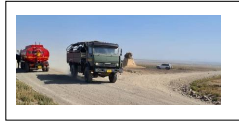
Figure 27: Rehabilitated Road at NCAA
