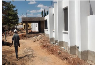
Figure 7: Construction of Maternity Block at Tabora RRH
