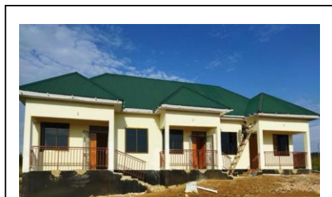
Figure 13 Staff house - Bukoba hospital
