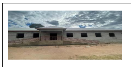
Figure 20: Dormitory for students with special needs at Masasi District (finalization stage)
