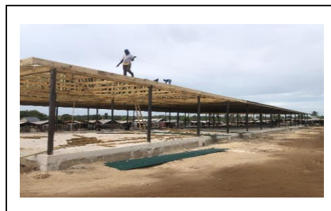
Figure 32: Construction of Bunju B Machinga Market in Dar es Salaam
