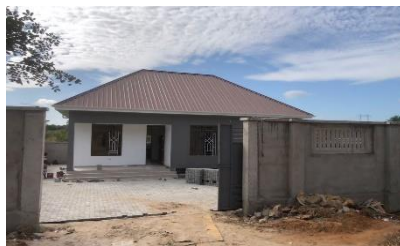
Figure 8: Construction of staff houses at Tumbi RRH
