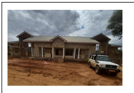
Figure 25: Mkomazi complex gate
